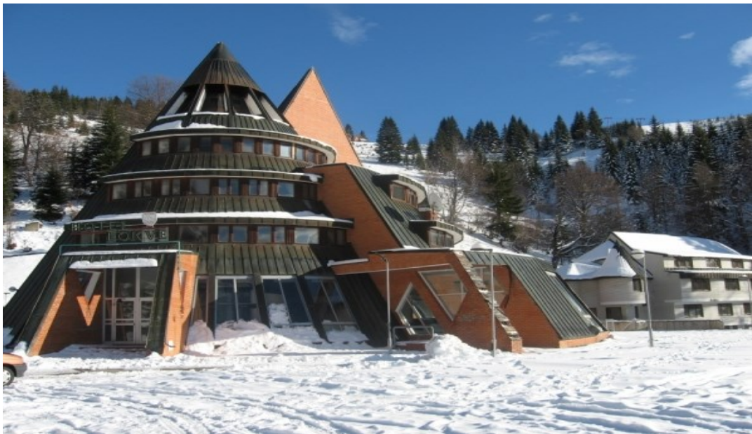
Figure 3. On the mountain Cmiljevica - findings the ski Center Lokve [25].
