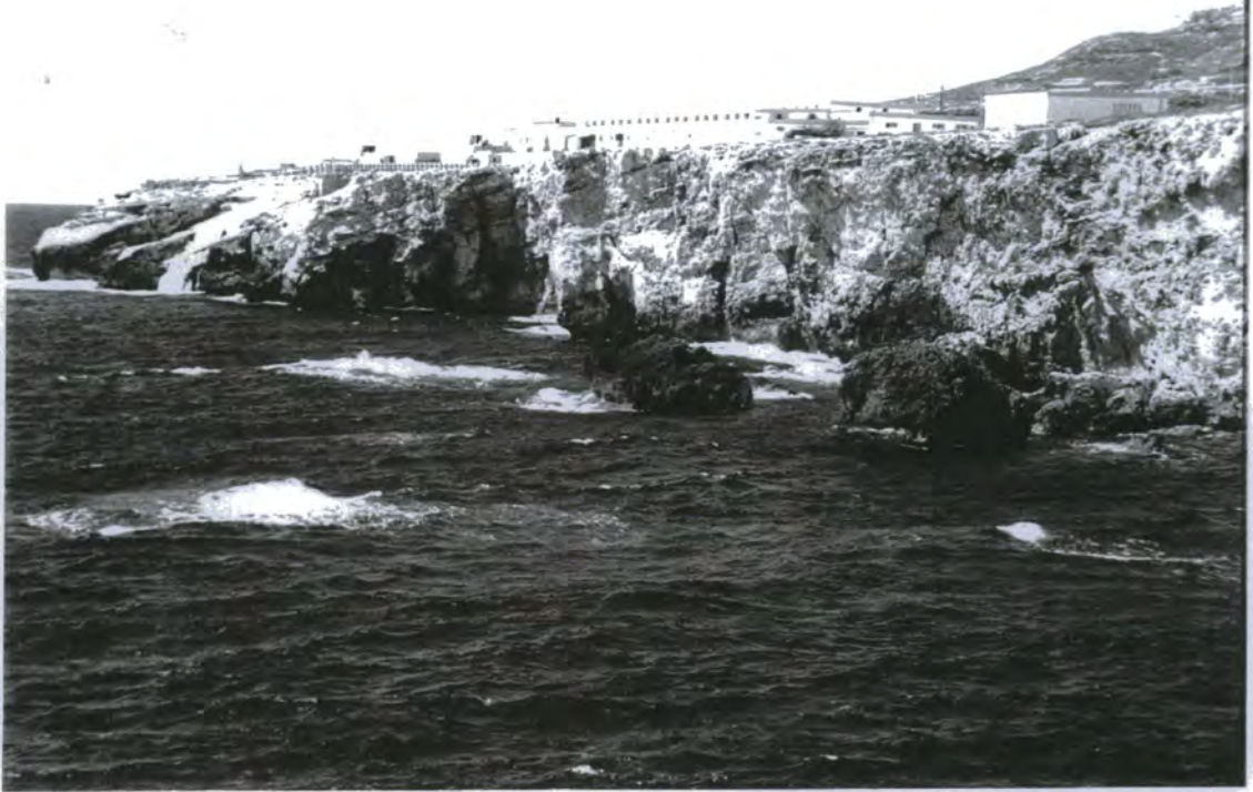
Plate 3.5. The Ghar Lapsi RO plant.
