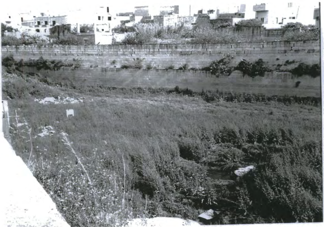
Plate 5.14. Accumulated rubbish (background) in a disused open reservoir.
