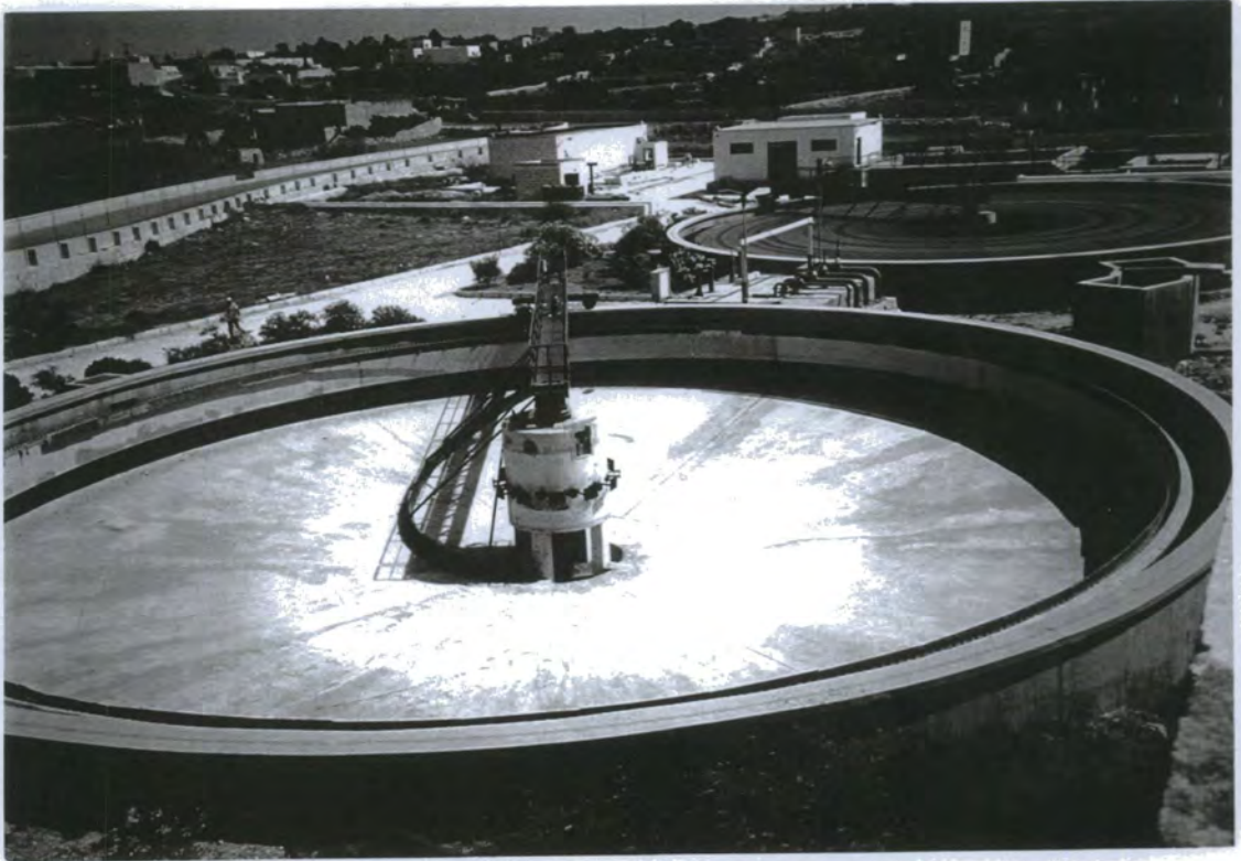
Plate 3.22. The Sant' Antnin Sewage Treatment Plant.
