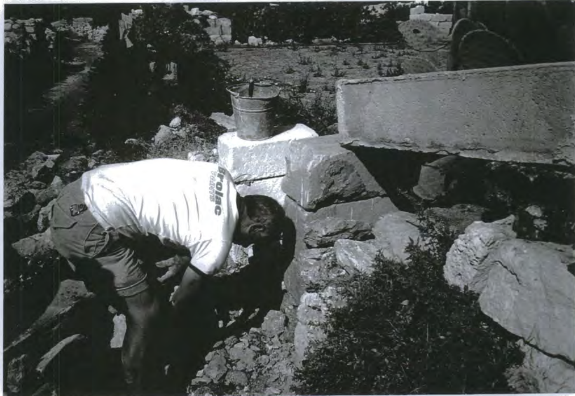
Plate 5.9. Workmen repairing a collapsed channel.
