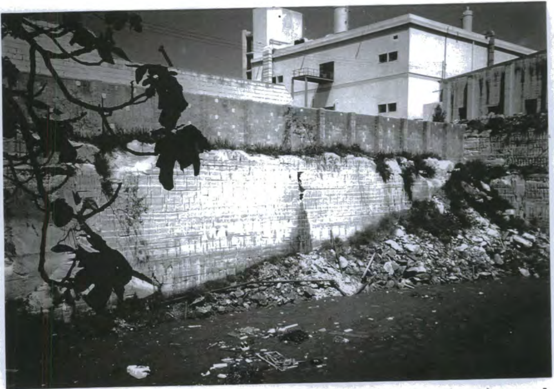
Plate 5.13. Waste from the SGS-THOMSON factory is disposed of in a disused quarry.
