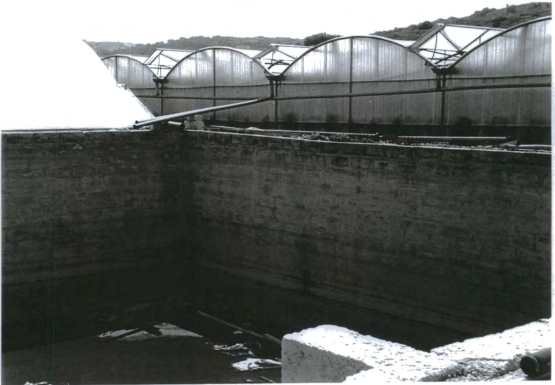
Plate 3.8. Rainwater harvesting from glasshouse roofs into a reservoir.
