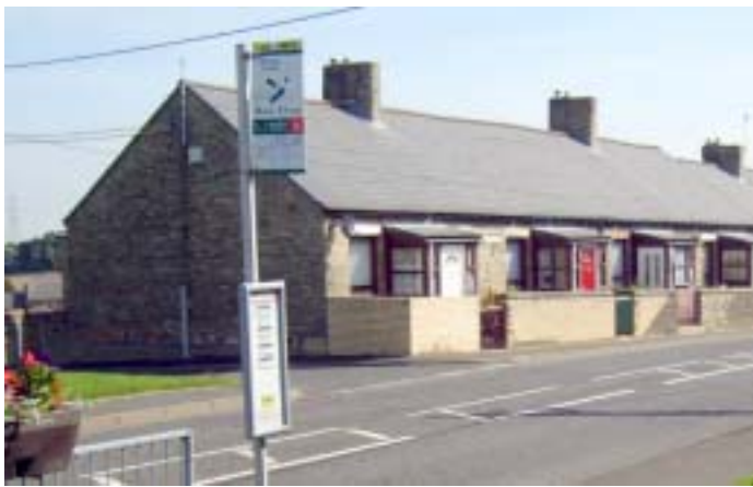
Howard Terrace - High Spen View of Howard Terrace showing the street frontage. The porches are modern. The roof-line is original.
