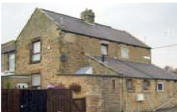
West Street - High Spen View of end-houses at right- angles to remainder of street. The offshot extensions are original although modified with small windows. The roof-line is original.
