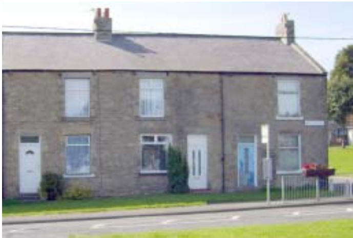
East Street - High Spen View from Howard Terrace showing the street frontage. The windows and doors are modern but the apertures are unmodified. The roof-line is original.
