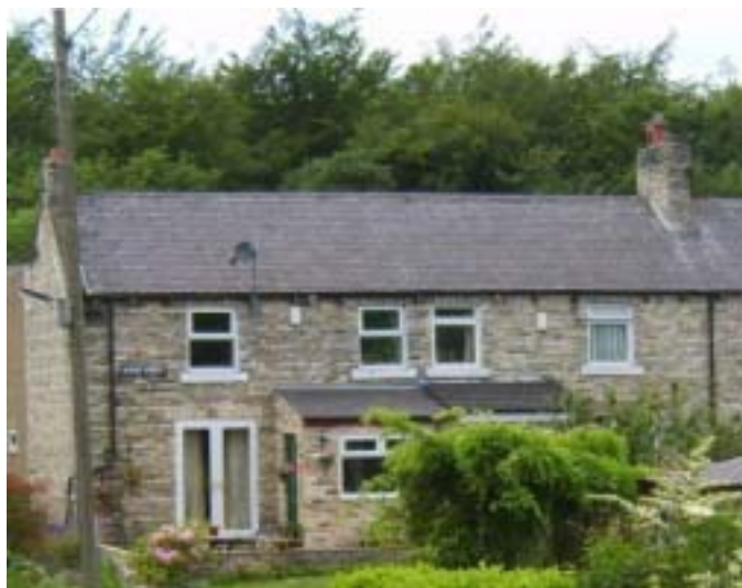
Albert Street - Victoria Garesfield View of house front. the small offshot extensions are additions. The French Window on the left was originally a window The original roof-line with slate roof is intact.
