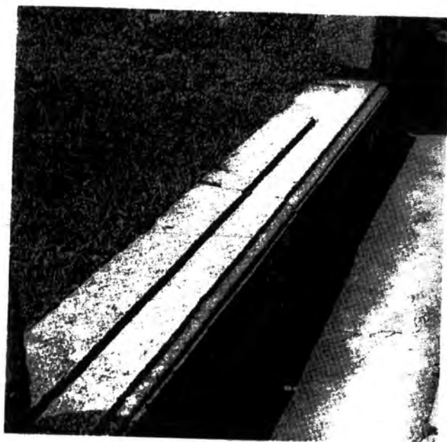
b. Groove for fixing a shop shutter (VII.12.11), Pompeii.
