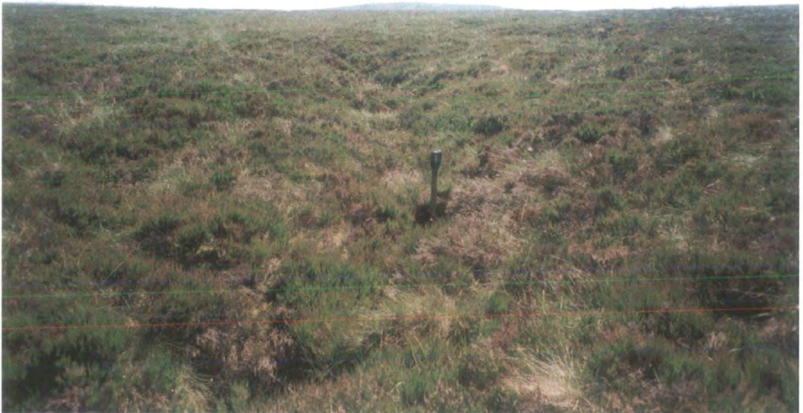
Figure 7.8. Surface depressions following the route of pipe 11.
