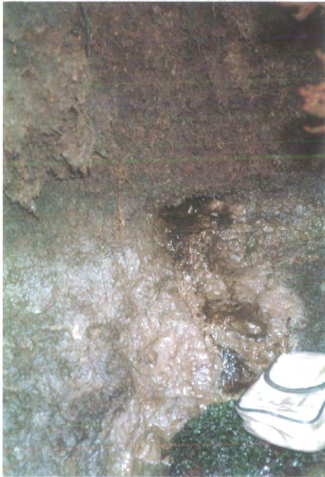
Figure 7.11. Example pipe outlets. a) Vertically elongated pipe outlet entirely within the peat. Note the mineral sediment on the floor of the outlet indicating upslope pipe contact with the mineral substrate. b) Horizontally elongated pipe at the peat-clay interface.
