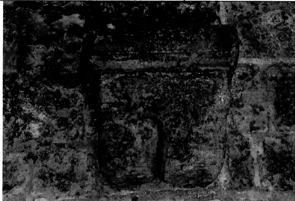
Plate 26 A Corbel Supporting the Intermediate Arch Within the Gatehouse at Prudhoe Castle
