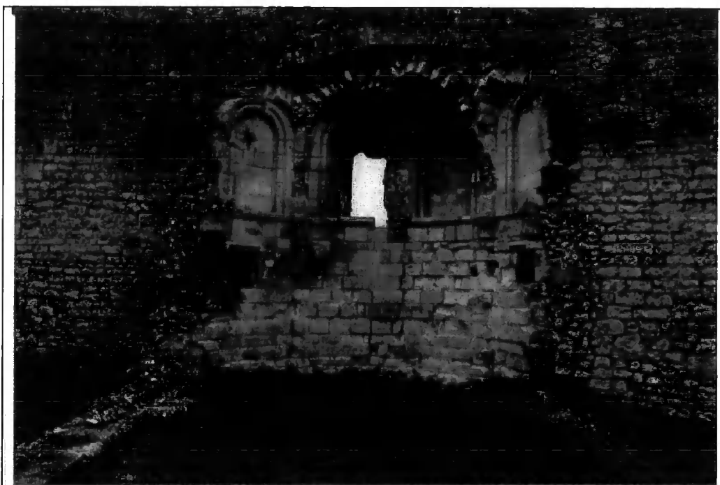
Plate 41 The remains of the chapel in the shell keep at Gisors Castle.
