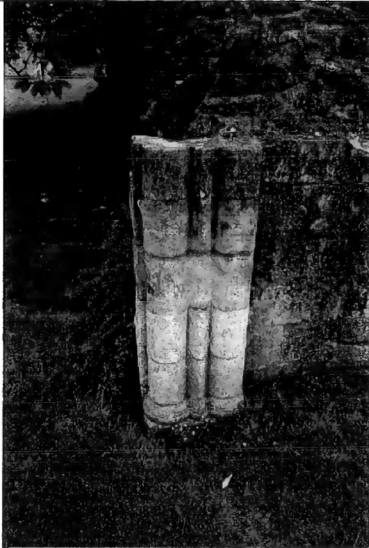
Plate 27 The Surviving Jamb of the Door from the First Church at Kirkham Priory Leading into the Cloister
