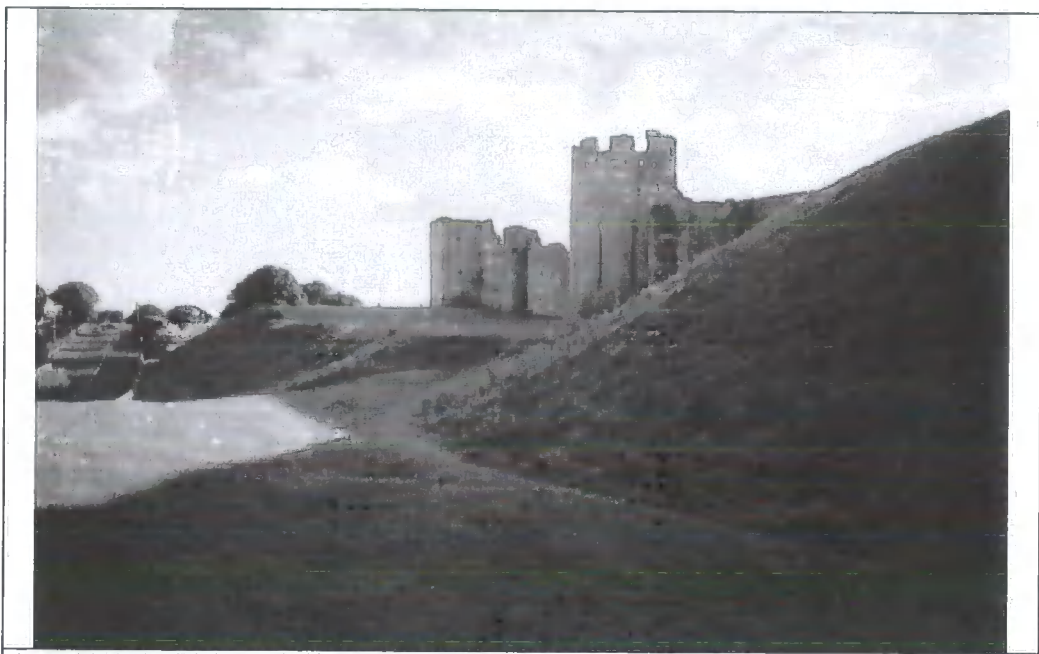
Plate 51 A general view of the south front of Warkworth Castle.
