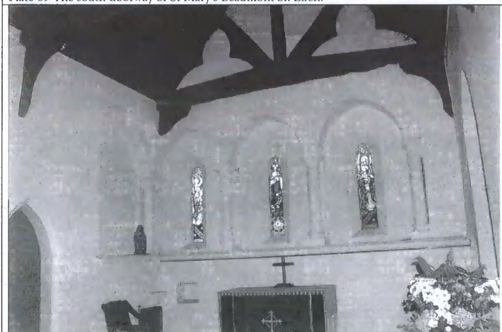
Plate 70 The arcading in the north and east walls of St Mary's Beaumont-on-Eden.
