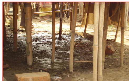
Figure 5.5: Waste disposal and urination practice underneath elevated houses
