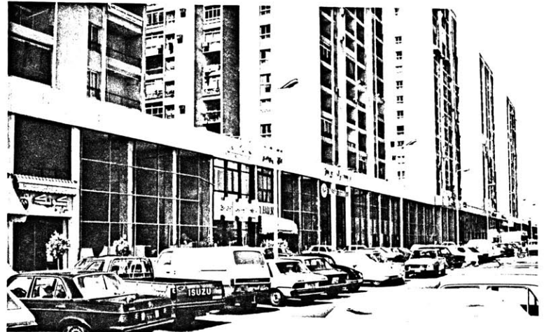
(13) Top, "temporary" shacks selling bread and essential groceries, near housing estate with no shops. Above, shops incorporated in other, more recent project.
