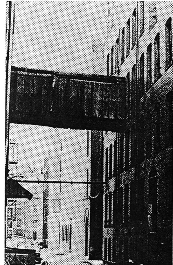
Fig. 2.5.4 Bridge connecting Fitz Shoe Factory and W.H. McElwain Company on Congress Street.
