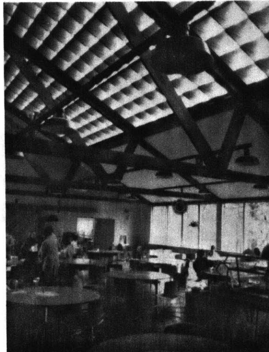
Skylights with reflective louvers allow winter sun to enter and block the summer sun. (Cambridge School in Weston, MA, Skylite concept by Norman Saunders, P.E.)
