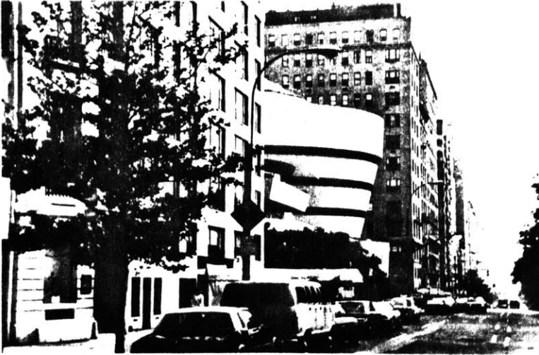
A major interruption in mass and detail, attracting attention and encouraging entrance.
