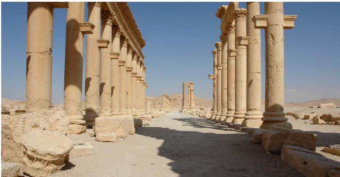
FIG. 94 Colonnaded street in Palmyra. The construction starts after the foundation as Roman colony in the mid 1st century A.D.
