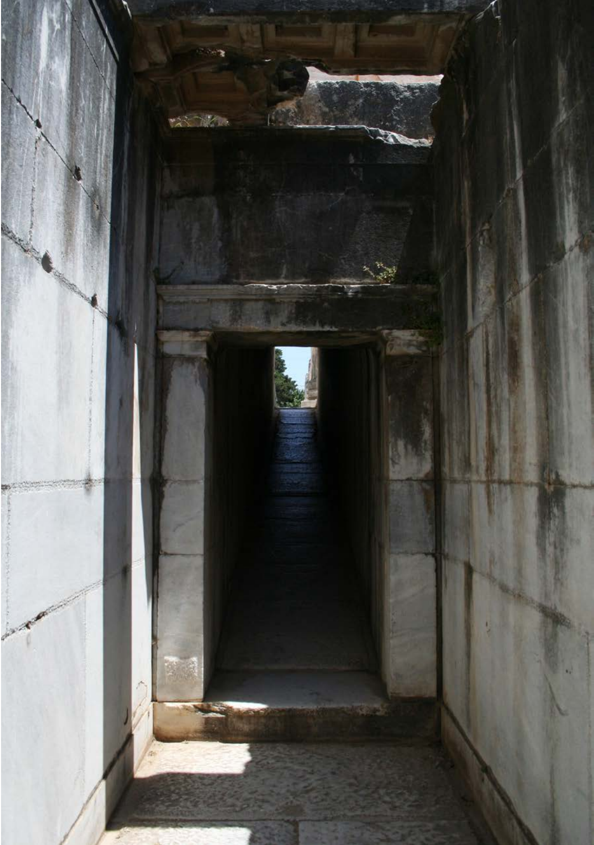
FIG. 59 View through the sloping tunnel which connects the internal court and the external world.
