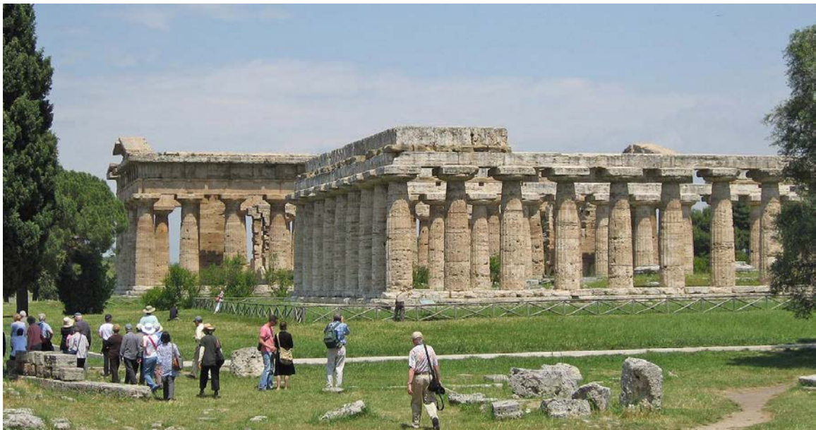
FIG. 36 Acropolis of Paestum in southern Italy: the two temples are juxtaposed . In front: Temple of Hera (basilica), 550 B.C, Behind it Temple of Neptune, 450 B.C.
