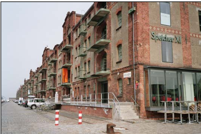
Fig. 17: Restored and re-used former storage buildings
