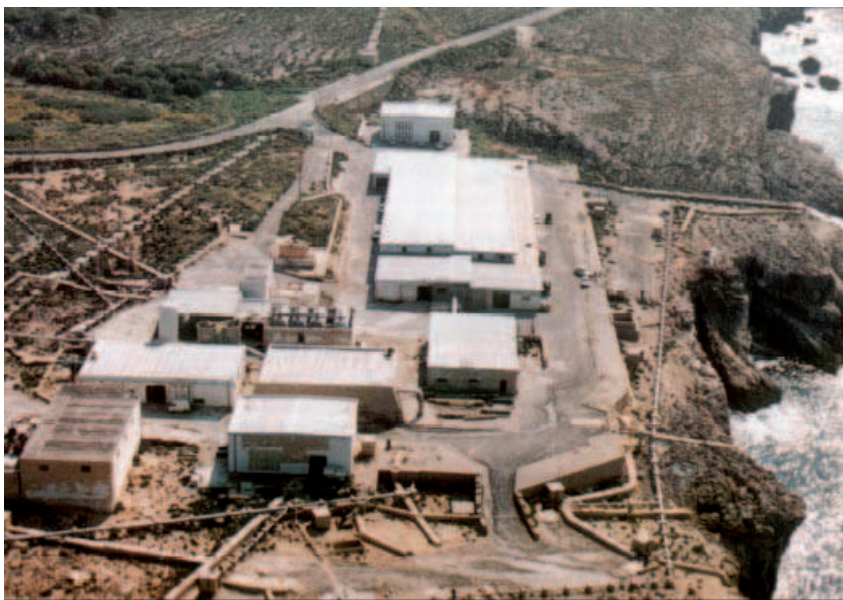
Figure 8. Reverse Osmosis Desalination Plant at Ghar Lapsi.
