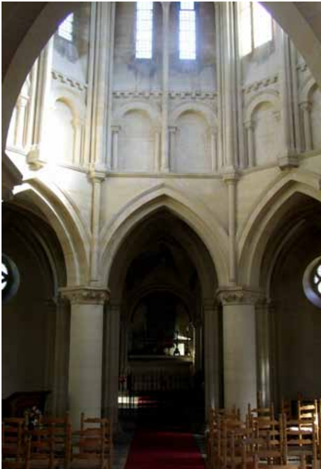
Fig. 9: Interior view of the chapel
