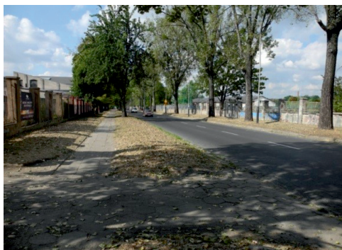
Photo 2. Section of the Milionowa Street over the Jasień river in subterranean canal
