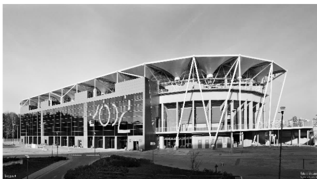
Photo 3. ŁKS City stadium (under construction) Source: http://fotopolska.eu/stadiony
