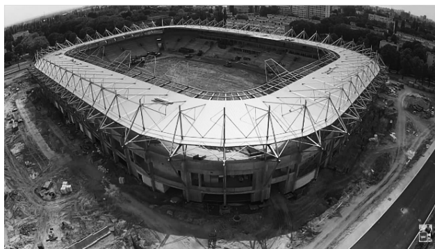
Photo 4. Widzew City stadium (under construction) Source: https://www.youtube.com
