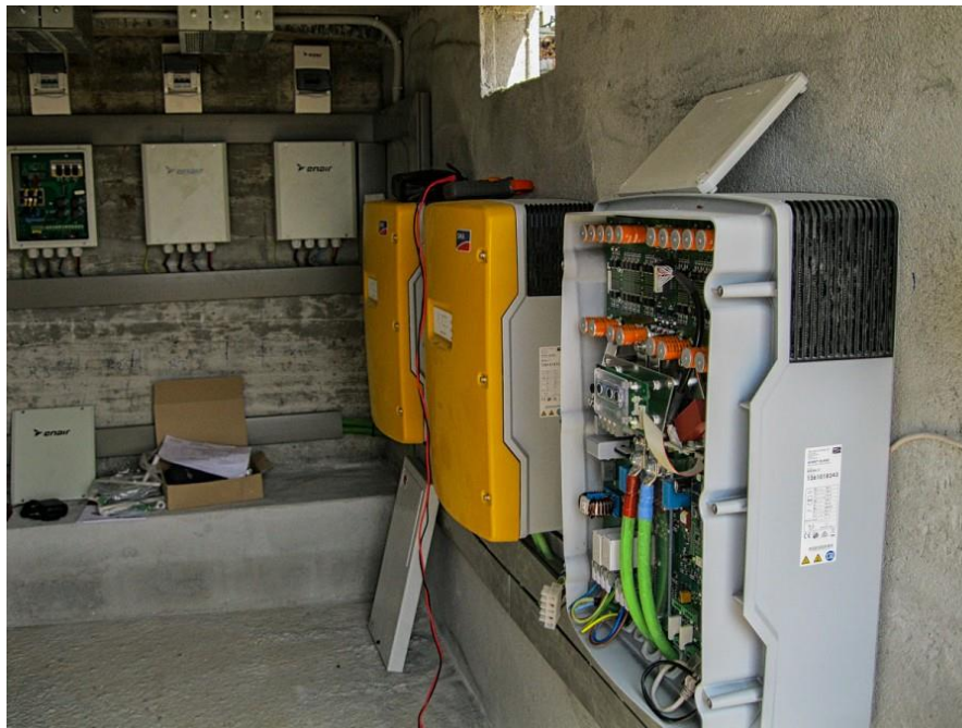
Figure 9. Installed inverters
