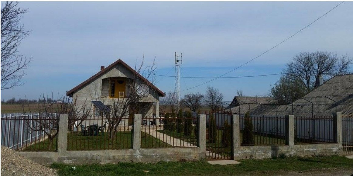
Figure 15. Wind hybrid power system in village Totoesti, county Iasi, Romania
