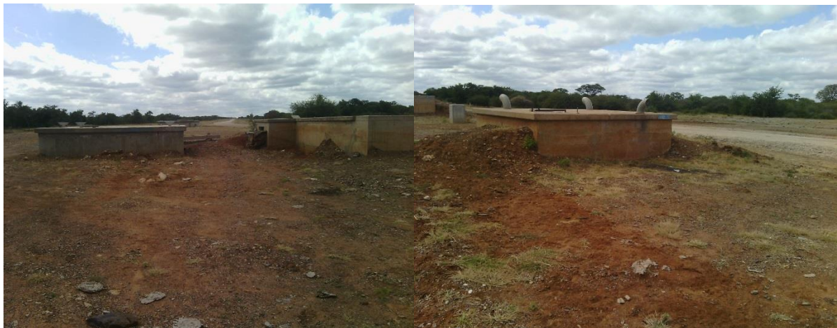
Figure 4.1: The NSC I pipeline near Palapye. Source: the researcher.
