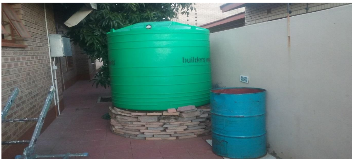
Figure 5.3: Showing a jojo tank (green tank) used to store water. Jojo is the trade name for a common brand of polythene storage tanks manufactured in South Africa. Source: the researcher.
