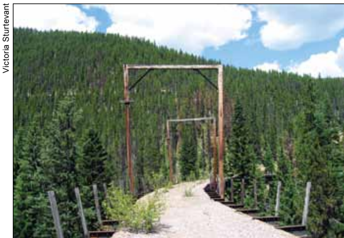
Figure 7-2—Abandoned Dominion trestle.
