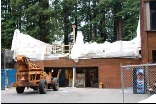
Figure 4-16—The Redwood Sciences Laboratory, Arcata, California, under construction.
