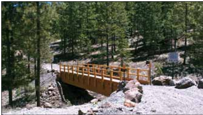
Figure 3-10—Saffel Canyon Trail Bridge on the Apache-Sitgreaves National Forest.
