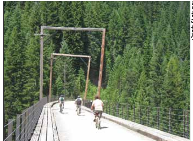
Figure 7-16—Bicyclists on the completed trail underneath catenary arches remaining from the old railroad. Catenary arches were used to hold electric wires powering the trains.
