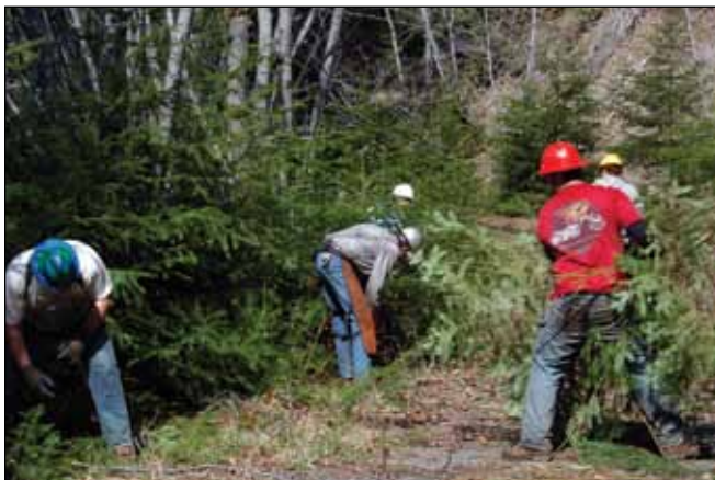
Figure 4-10—Removing roadside brush by hand.
