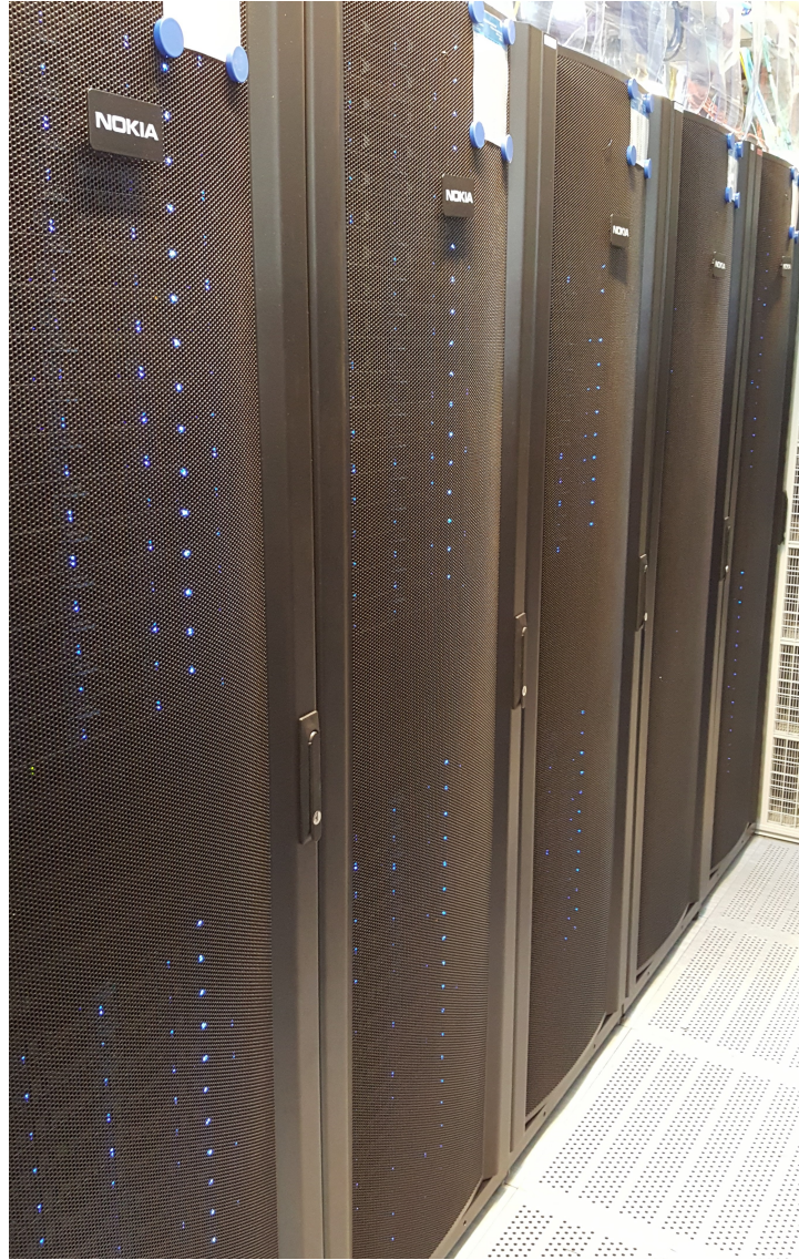
Figure 1: Data center cabinets, serving as physical mounting points for tens of servers.
