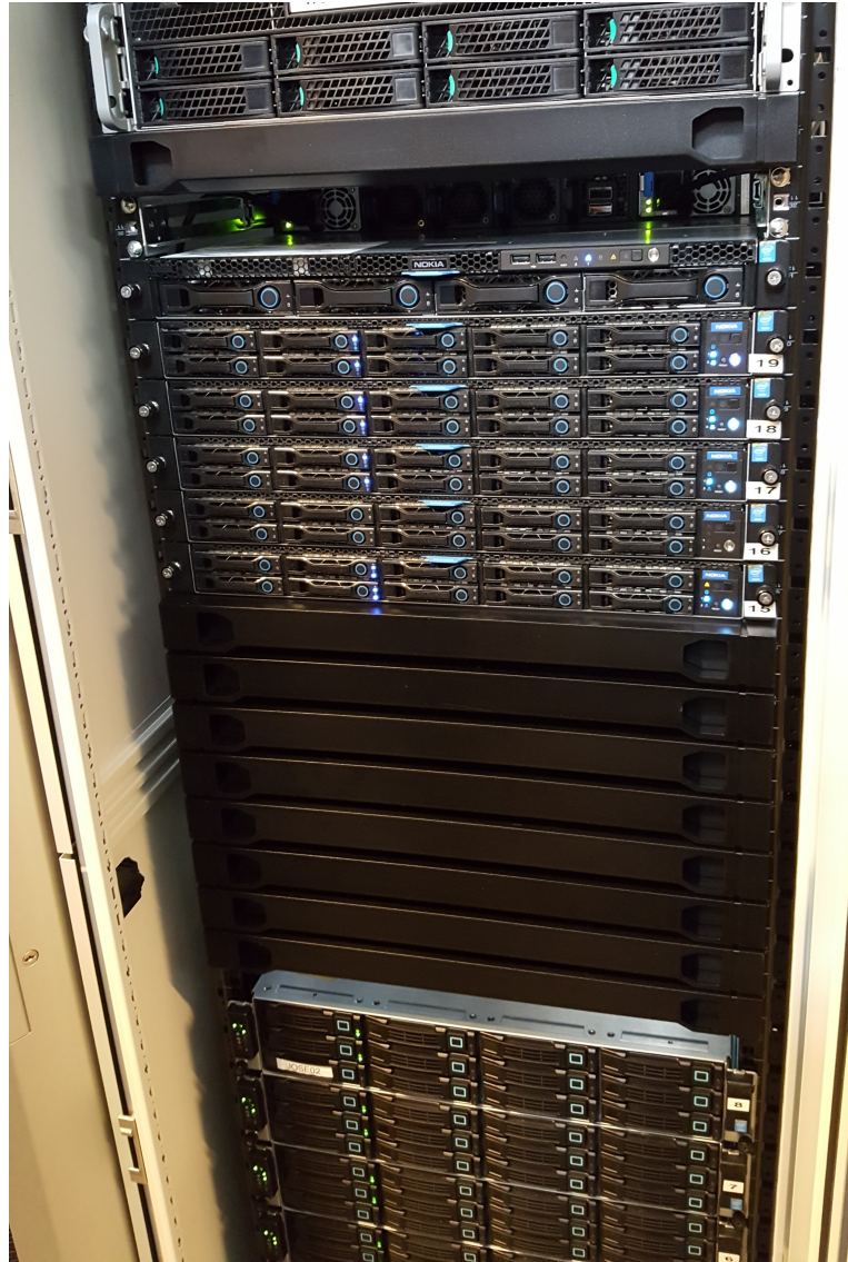
Figure 4: Server rack mounted inside data center cabinet. At least 8 different physical servers can be seen in this picture, as well as some empty slots.
