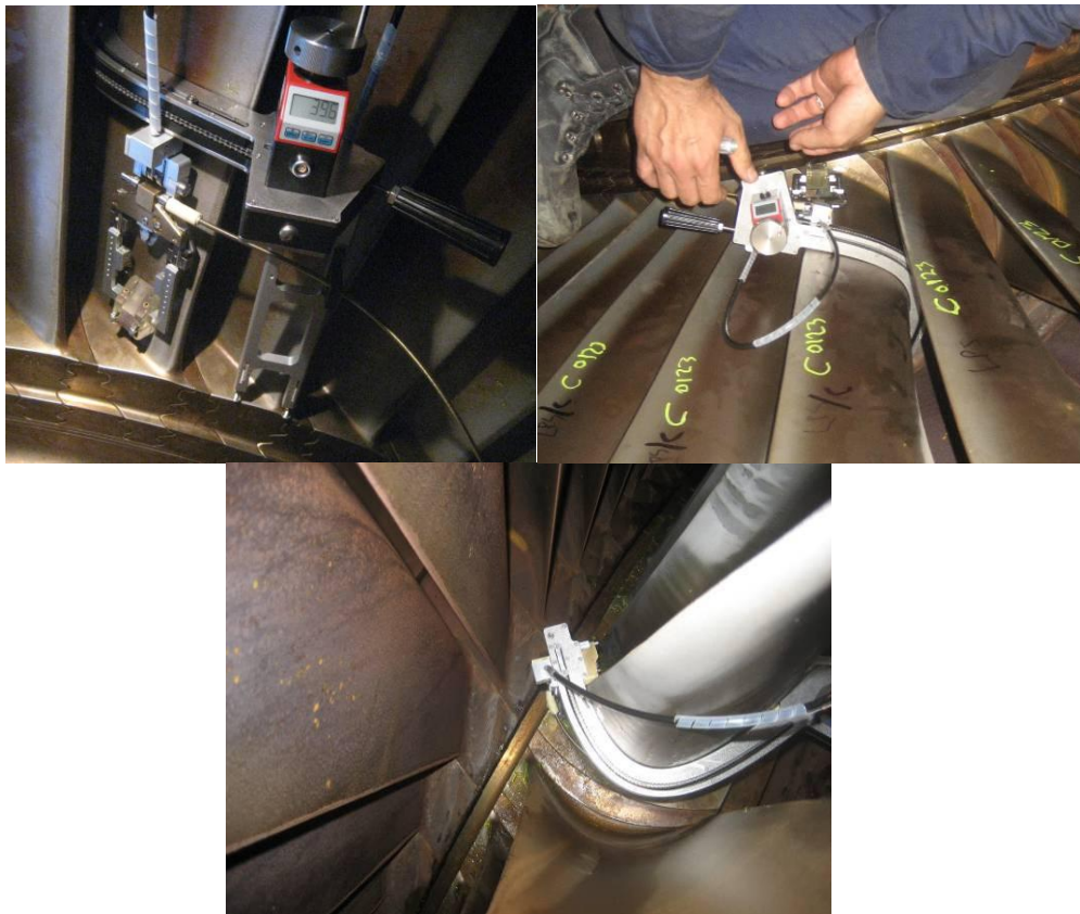
Figure 5-21 Images of scanning frame positioned on a rotor in-situ
