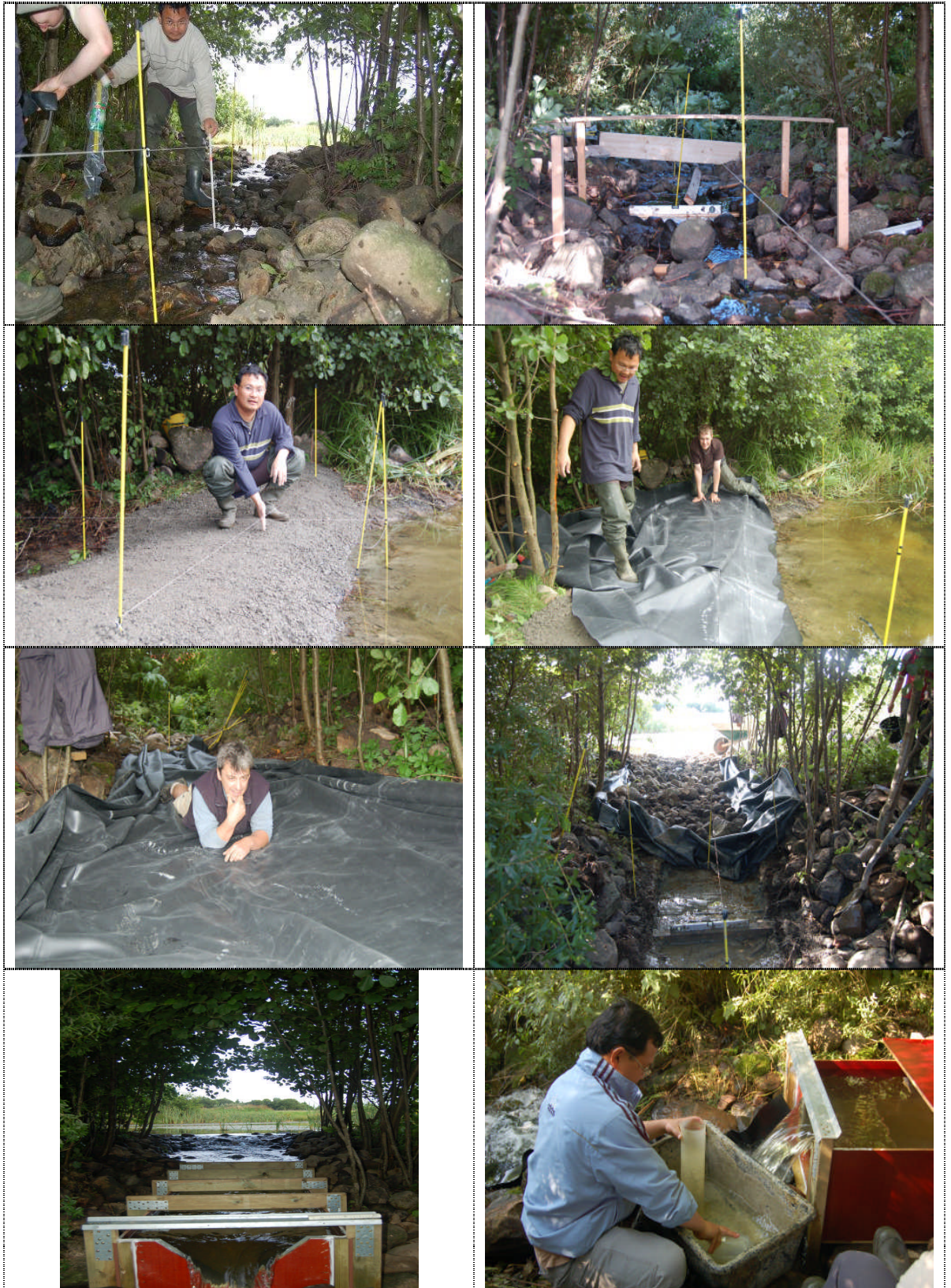
Figure 10-10. Pictures of preparation and construction of Lyby Field Flumes.
