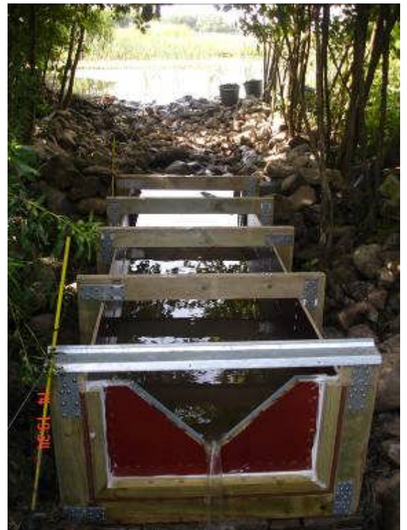
Figure 10-5. Constructed Flume at the outlet of third pond.
