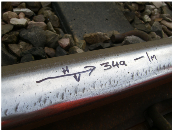
Fig. 2: RCF cracks on a rail
