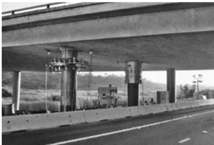
Fig. 2-1 The XXsys carbon fiber jacket site filament winding technique (USA) [9]
