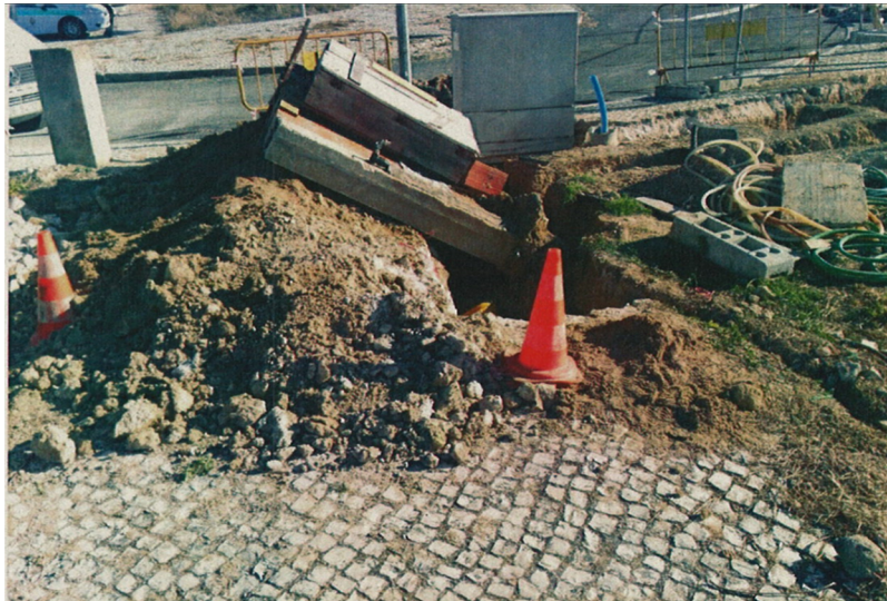
Fig. 1. Death scene demonstrating wall collapse.
