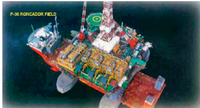
Sl.16 Naftna platforma
