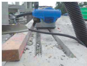
1. Cutting Grooves and Cleaning
