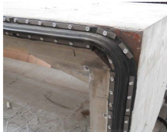
Fig. 5: Installation of the seal
