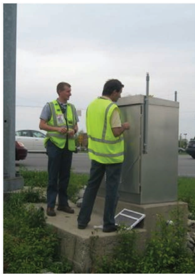
(a) Temporary "tie-wrap" station.
