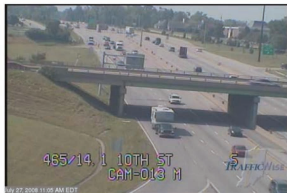
(d) 11:05 am. Northbound I-465 queue cleared; I-465 flow normalized and ramp reopened.
