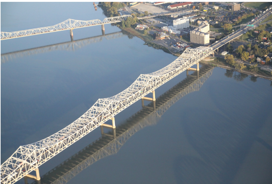
Top. Construction of new I-65 Ohio River Crossing (1962).
