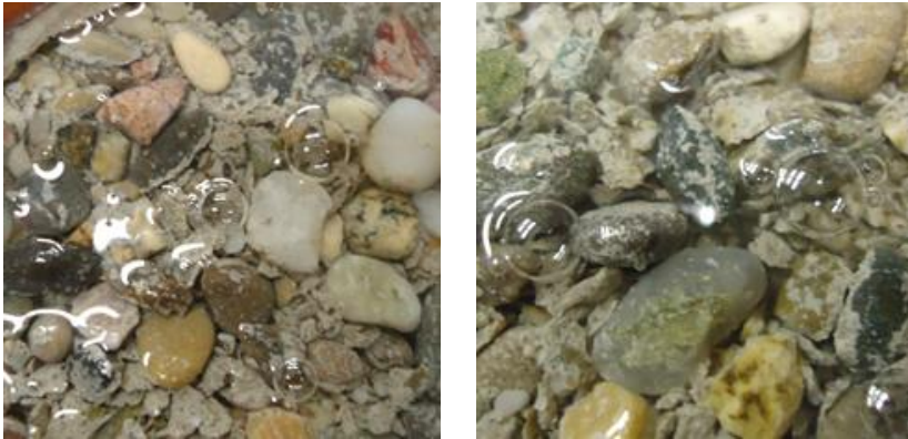
Figure 4-4: Loose fragment remains composed of exfoliating scales of cement paste, quartz gravel with little adherences of cement paste, and the presence of gas bubbles coming from the debris' interior, S70 by the end of the 56 days' cycle (CEN/TS 12390-9).
