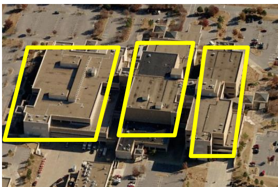
Figure 32: Additional surveyed facility building forms
