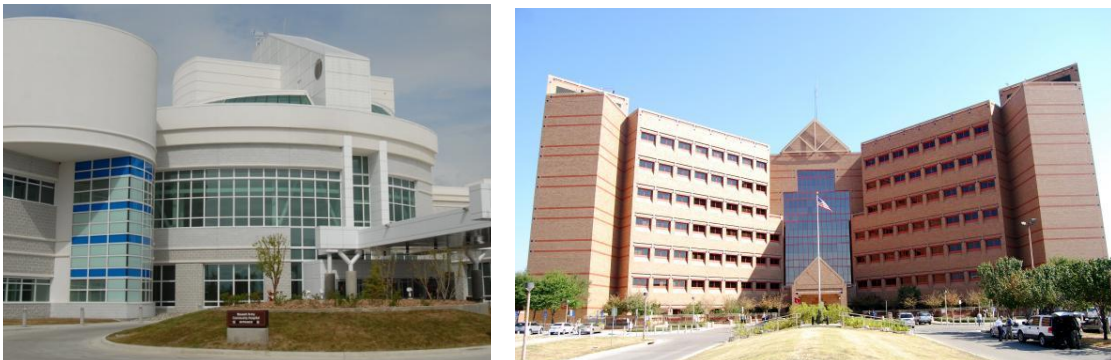
Figure 7: Selected facilities - Bassett Army Community Hospital, Fairbanks, Alaska; and Brooke Army Medical Center, San Antonio, Texas
