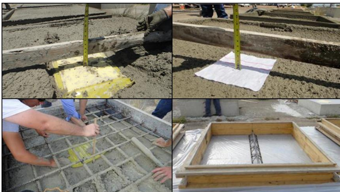
Fig. 3. Construction of slabs with simulated defects
