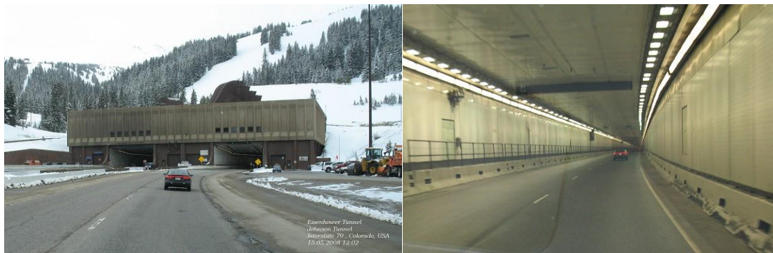
Fig. 24. Eisenhower Memorial Tunnel, CO. Photographed by Bernd Kramarczik, http://en.structurae.de/photos/index.cfm
