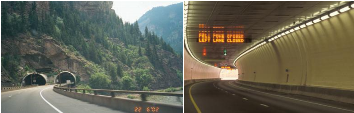
Fig. 31. Hanging Lake Tunnel: exterior (left, from http://www.mesalek.com/colo/glenwood/guide.html ) and interior view (right, FHWA, http://www.fhwa.dot.gov/publications/publicroads/04mar/04.cfm )
