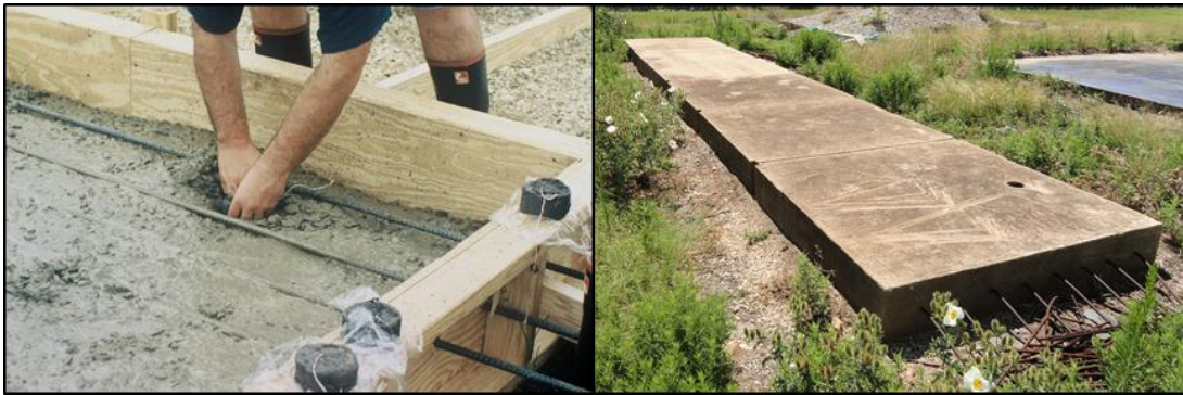
Fig. 7. Clay lump slab construction
