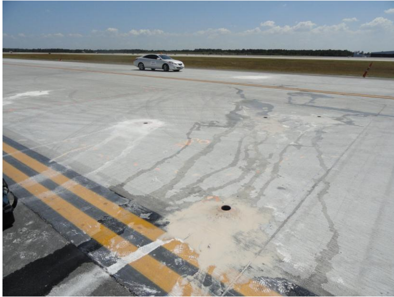
Fig. 60. Airport runway at IAH
