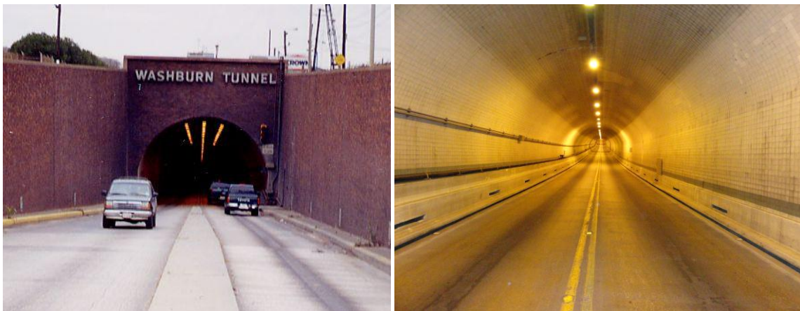
Fig. 52. Washburn Tunnel: exterior (left, from http://www.texasfreeway.com/houston/photos/around_houston/around_houston.shtml ) and interior view (right)
