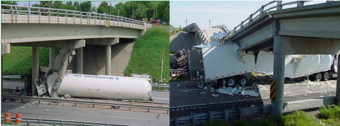
Fig. 1.2. (Left) Collision of truck with bridge column (Staples, 2007); (Right) Collapse of bridge on I-80 in Nebraska after being struck by a tractor trailer (El-Tawil et al., 2005).
