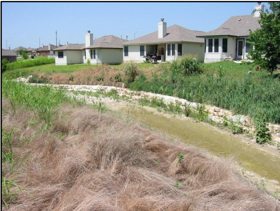
Figure 5. After stream restoration in 2008 (City of Austin).
