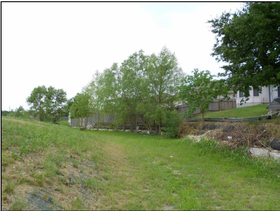
Figure A-18. Walnut Creek at Ritchie Drive after restoration in May 2011.
