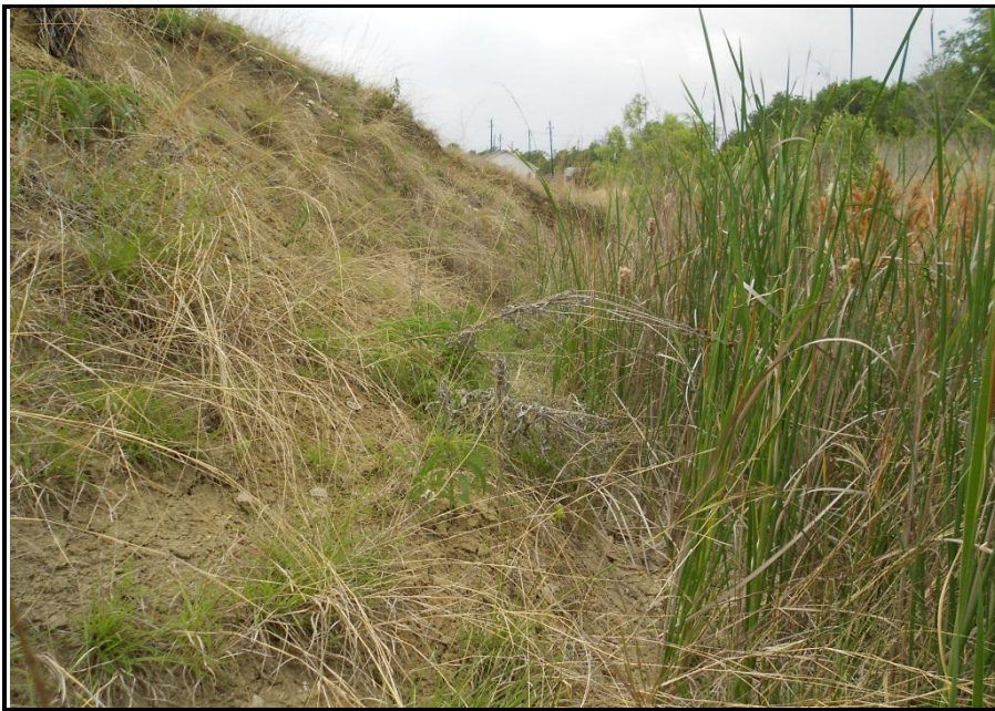
Figure A-10. Walnut Creek at Ritchie Drive after restoration in May 2011.
