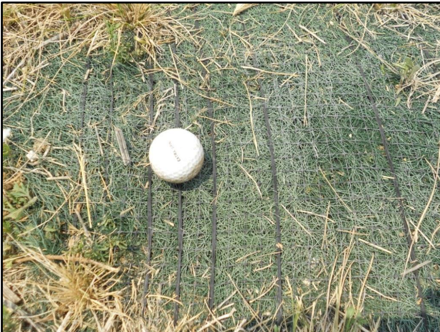
Figure 7. Vinyl netting to minimize erosion problem.
