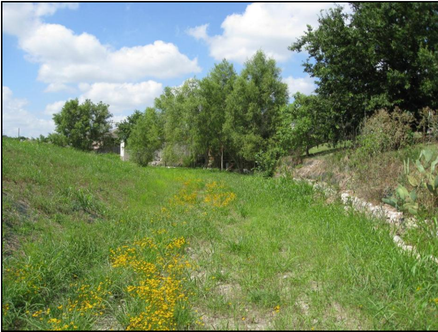
Figure A-17. Walnut Creek at Ritchie Drive after restoration in June 2010 (City of Austin, 2010).
