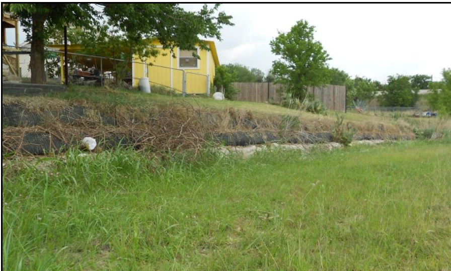
Figure A-12. Walnut Creek at Ritchie Drive after restoration in May 2011.
