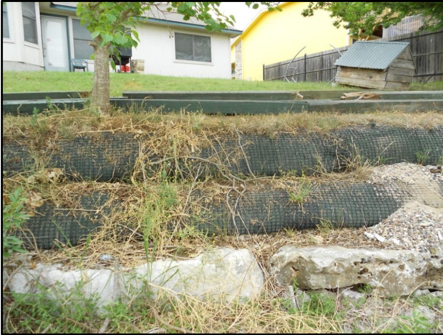
Figure 6. The bank was stabilized with rocks, vegetative layers, and soils.
