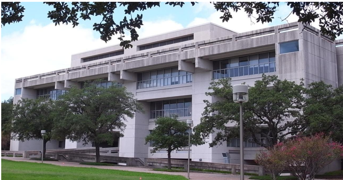
Figure 13. Langford Building A from the Front
