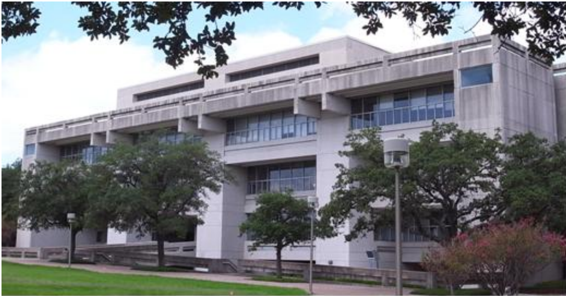
Figure 1. Langford Building A Façade
