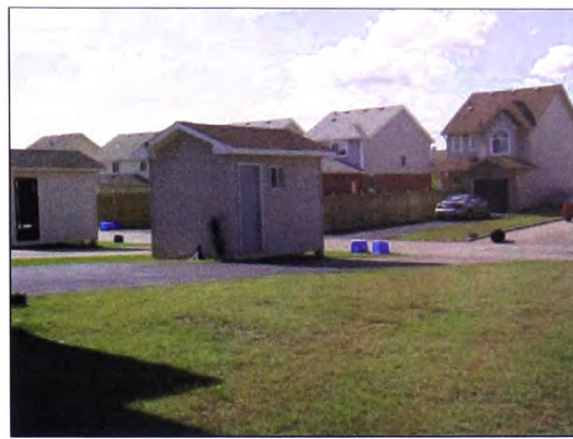
Figure 4.12: Rear streetscape depicting mix of garage/storage options
