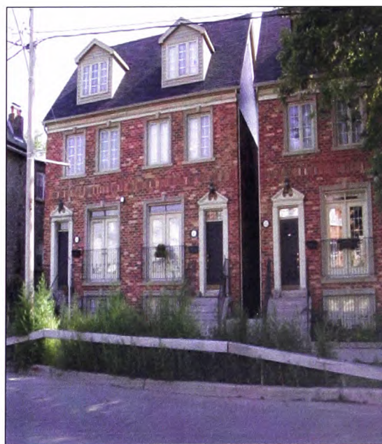
Figure 5.2: Toronto semi-detached infill in vicinity of The Beach
