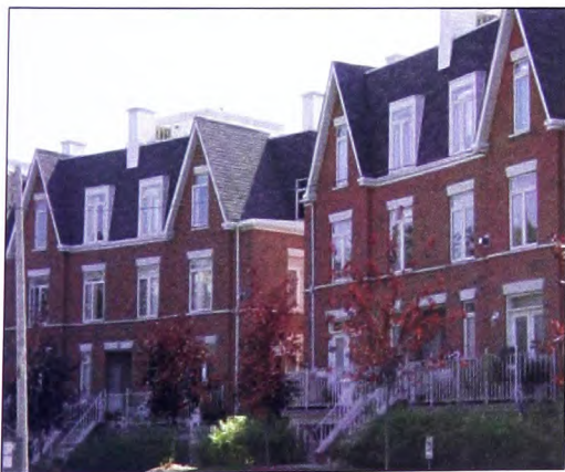
Figure 4.19: Stacked townhouse condominium units
