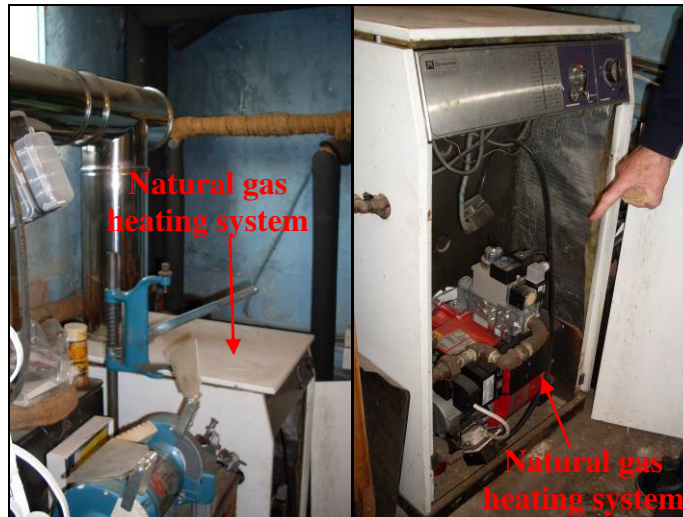
Figure 5-8: Natural gas heating system (type SPG 146 – 1, 23.5 to 85 kW capacities)
