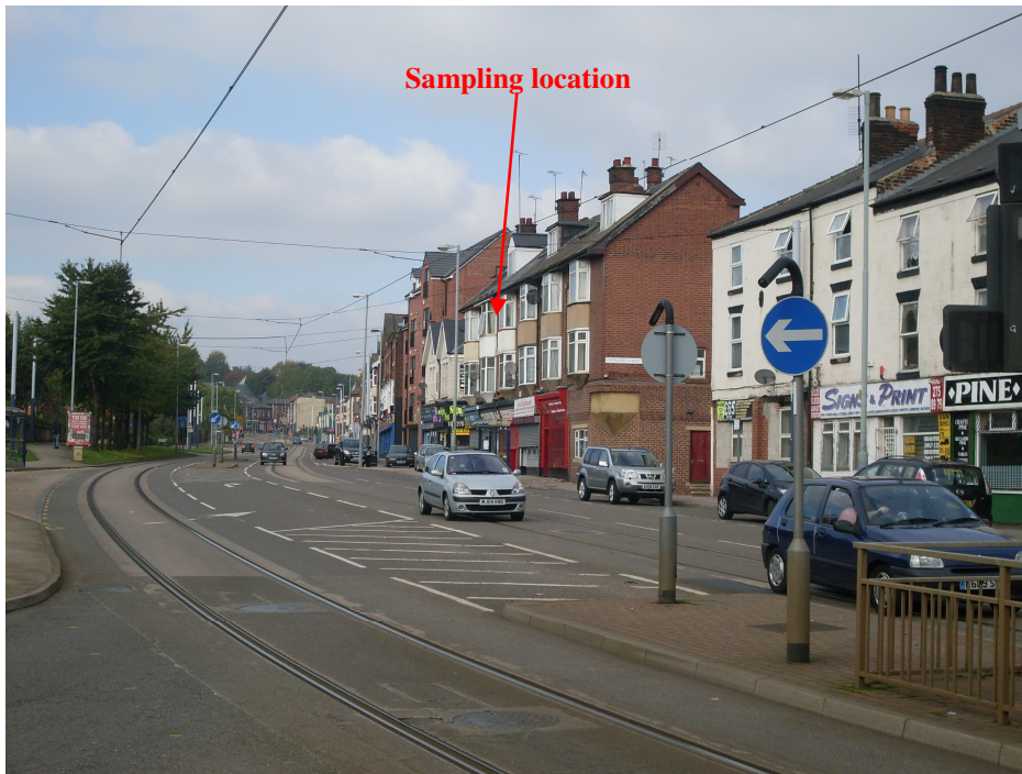
Figure 7-3: Street view of the residential flat for Case 3
