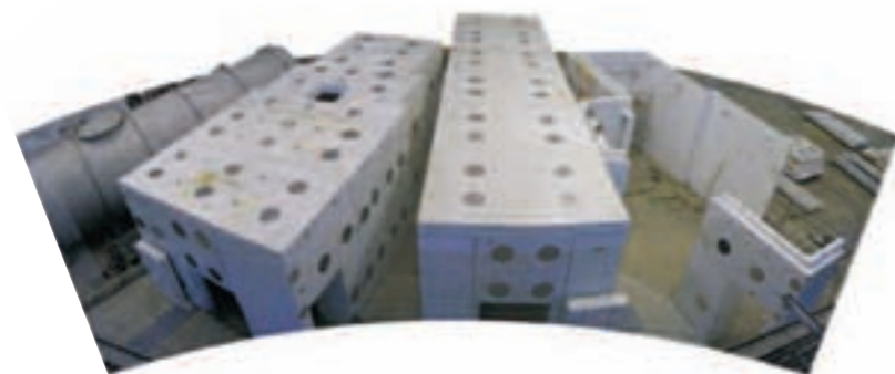
From left to right: the SANS2d vacuum tank, blockhouses in grey undercoat for the Polref, Inter and Offspec reflectometers (25th May 2007).
