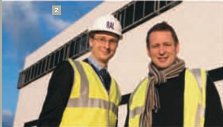
2. Rt Hon Ed Vaizey, MP, seeing the ISIS Second Target Station project in February. Jonathan Carkeet, TS-2 installation task leader, is showing him round. 07EC1279
