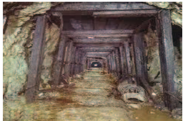
Figure 3. Timbering in tunnels.
