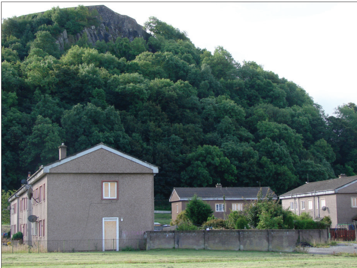
Photograph 3 Raploch Orlit housing, Glendevon awaiting demolition, 2007
