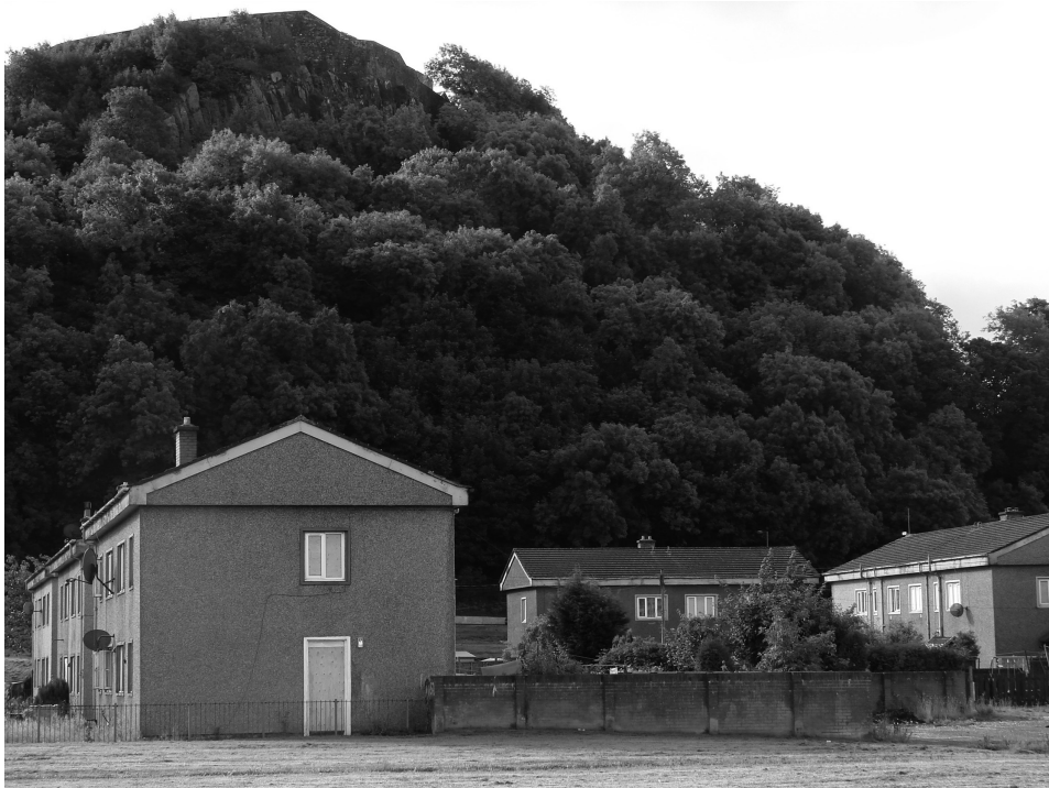
5.4 Raploch Orilt housing, Glendevon awaiting demolition, 2007 (Source: Douglas Robertson)
