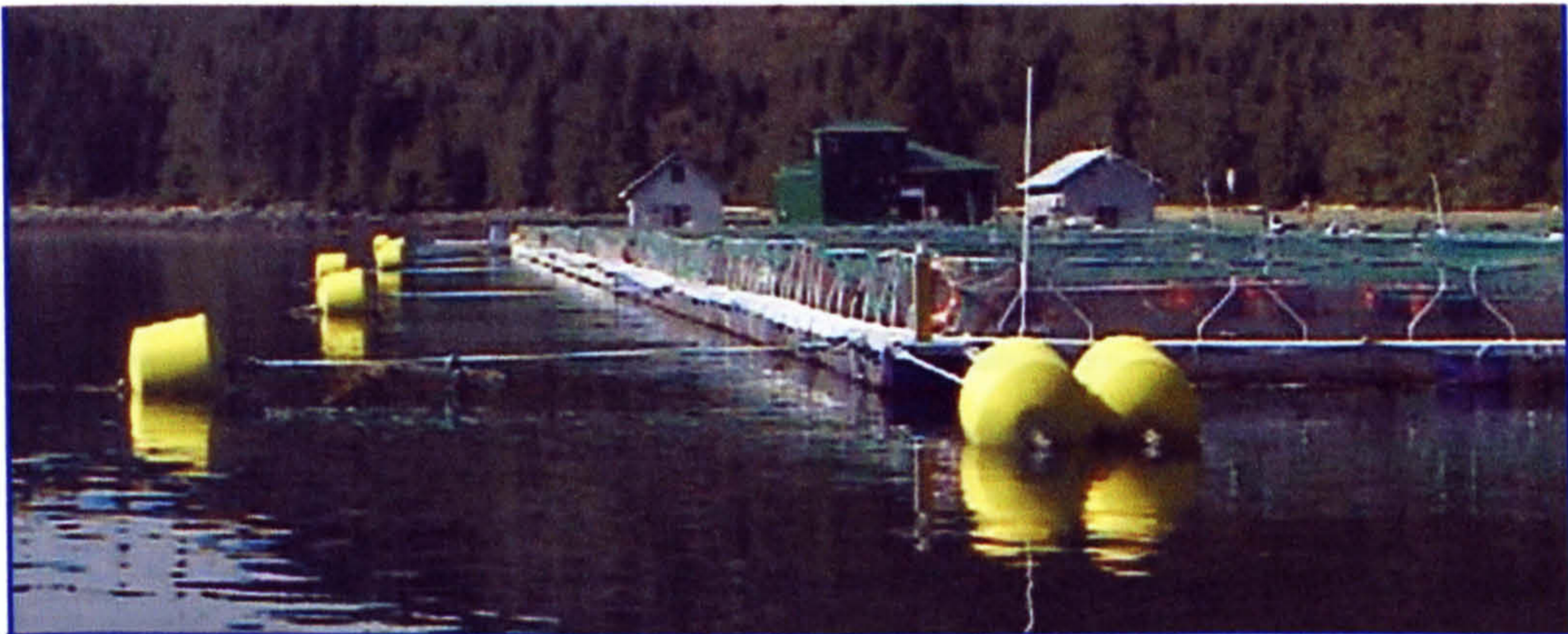
Figure 17: Surface view of Venture Point farm site (looking southwest). Twin anchor lines, shown in the foreground, secure the system against the strong tidal flows characteristic of this site. A feed shed (center) and site accommodation are indicated at the opposite end of system.
