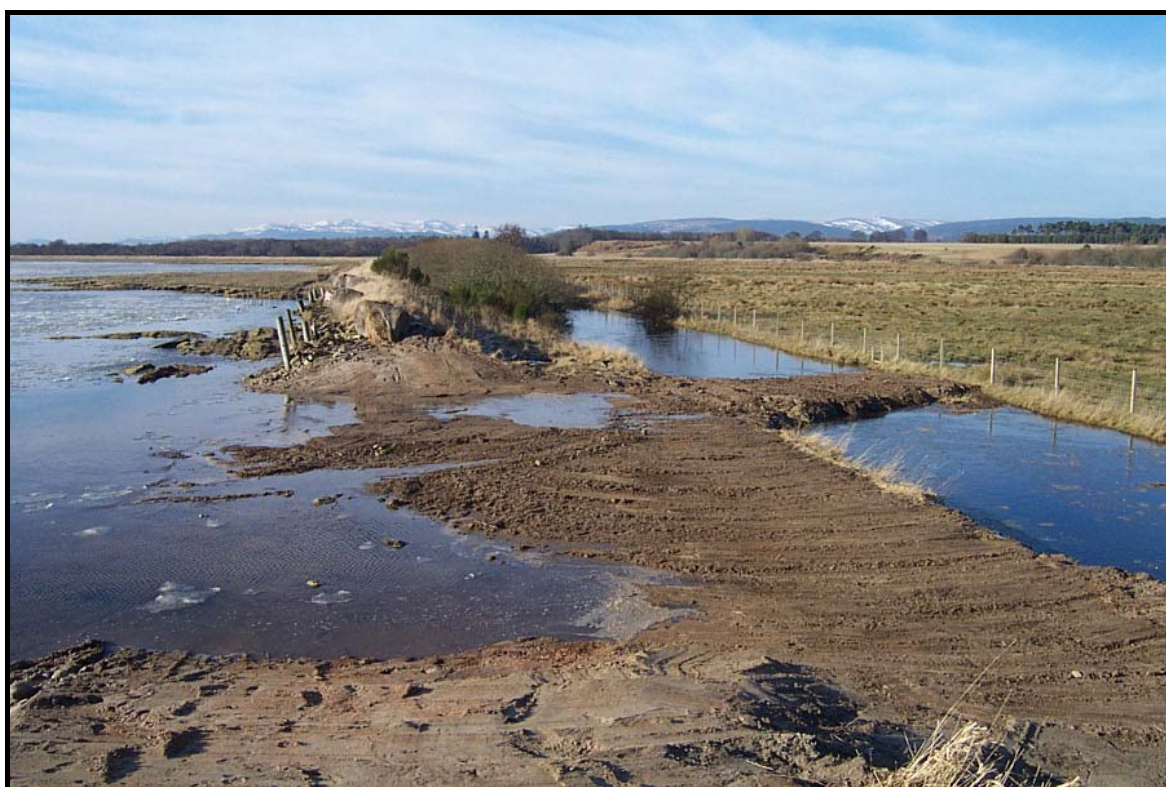
Figure 2.6: The first tide that entered Nigg Bay Managed Realignment Site following breaching. View looking along the southern embankment across the east breach gap, with Nigg Bay to the left and Nigg Bay Managed Realignment Site to the right. RSPB.
