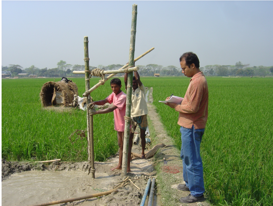
Observation on the installation of a shallow irrigation pump in ricefield.
