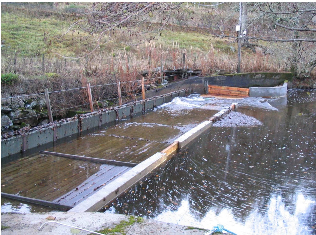
Figure 2.4 The downstream trap at Girnock Burn. Only the 'sieve' at the end furthest from the viewer is in action.
