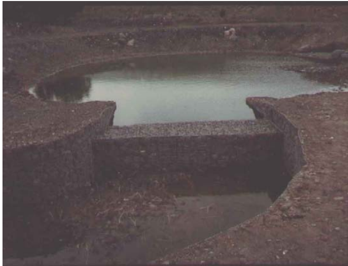
Plate 7.12 The collection pond of the 'treatment plant'
