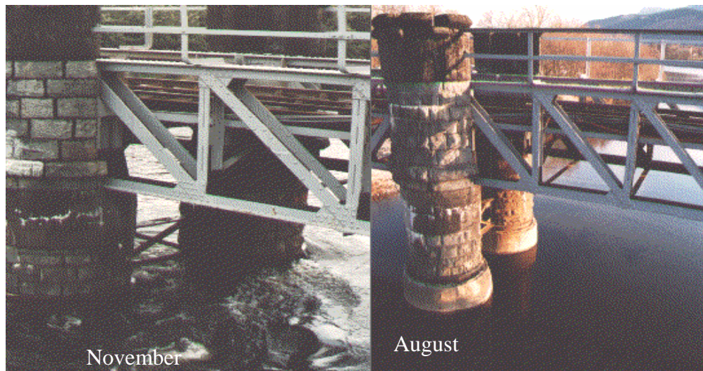
Plate 7.3 Comparison of river levels in August and November at the Lochy Viaduct
