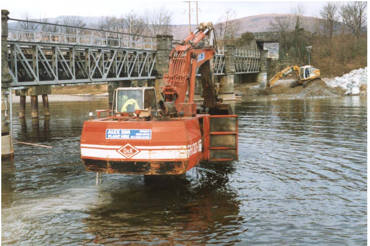
Plate 7.9 Excavator finally underway
