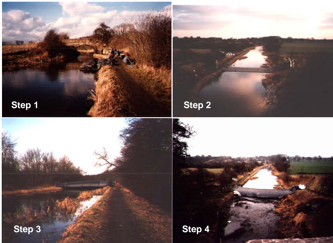
Plate 7.11 The sequence in the utilisation of the portable dam
