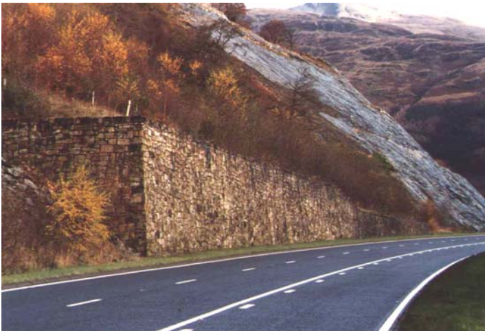
Plate 7.2 A82 Landslide prevention project
