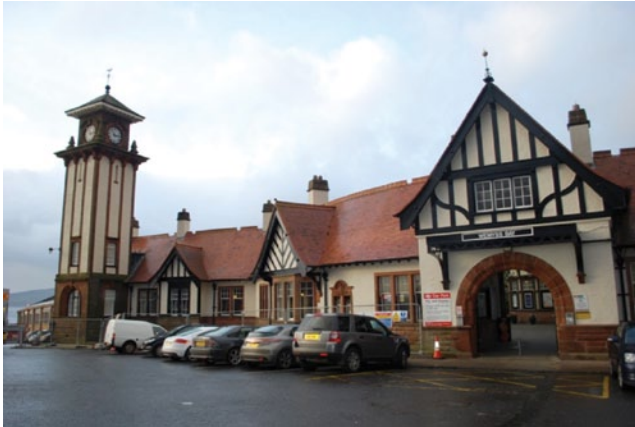
Refurbished Exterior at Wemyss Bay
