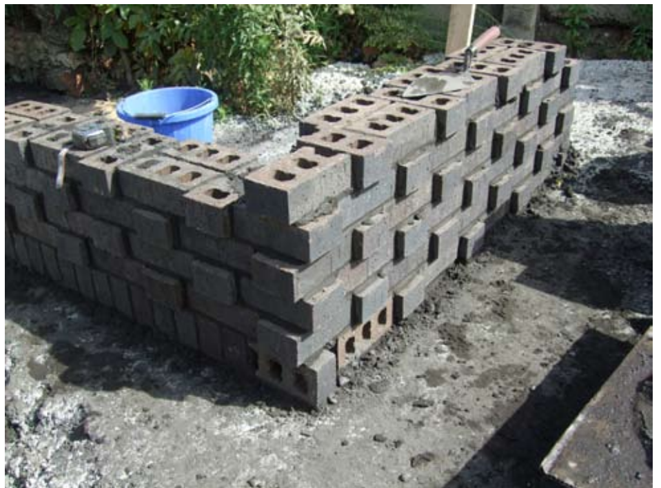
Brickwork Sample Panels
