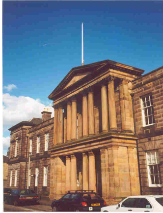
Figure 5: Edinburgh Geographical Institute in Duncan Street, Edinburgh. Falcon Hall was demolished in 1909, but an idea of its grandeur can be gained from its classical portico, which was rescued and now fronts the EGI building above.
